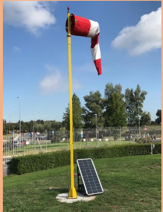
ON FIELD INSTALLATION (ROME)
